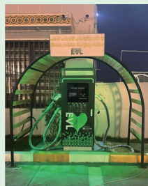
600KW Charging stack with 8 guns for E-truck
